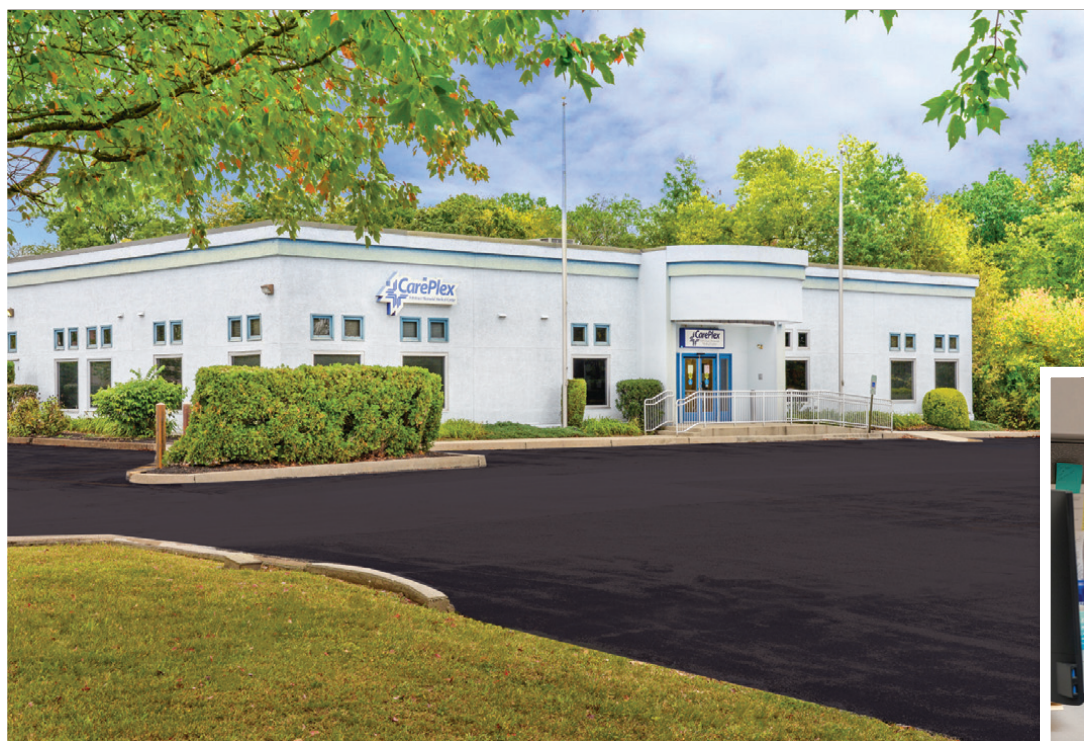
Occupational Health is part of the Pottstown Hospital CarePlex building located at 81 Robinson Street, Pottstown.
