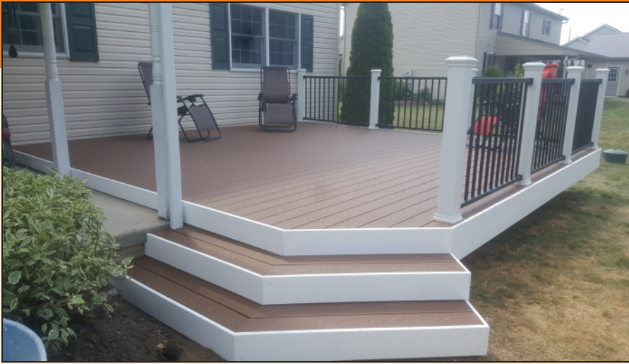
Trex Deck with reveal Railing system constructed by HOMEWERKS LLC.
