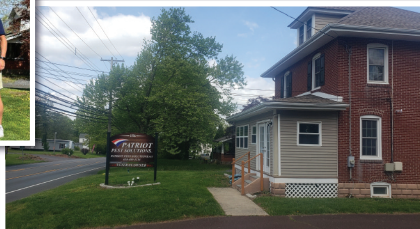
The new Patriot Pest Solutions office located in Limerick
