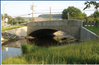
Bridge Replacement Berks County, PA
