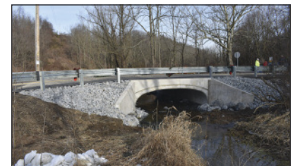
Emergency bridge replacement.
